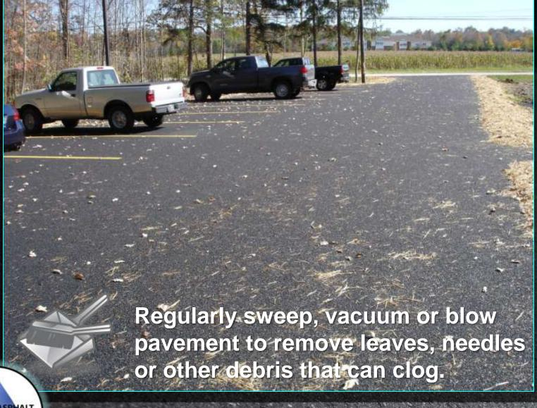
POROUS ASPHALT PAVEMENT
