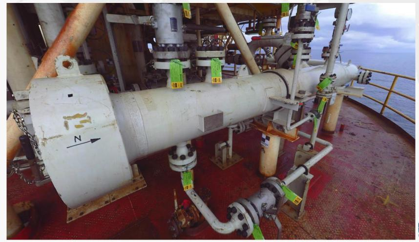
12" Main Production Pig Launcher- FPSO O3D Design
