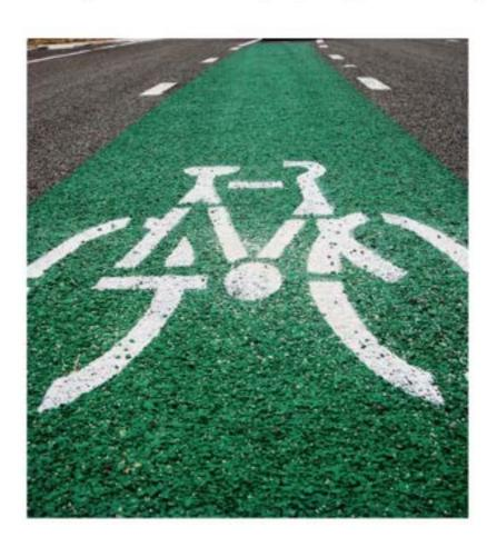
There is a growing awareness of the need for cycle safety on regional roads. Typically regional roads are constructed with a more coarse bitumen mix commonly known as spray seals. This has led to MPS adapting the product to meet these specific needs. The result has been excellent adhesion and flexibility on a wide variety of surfaces.
