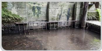
With minimal changes to the overall structure of the weir, the domestic supply to the cottages could be maintained whilst also complying to the abstraction conditions which were in place for the HEP licence, optimising the abstracted quantity and maximising power generation.
