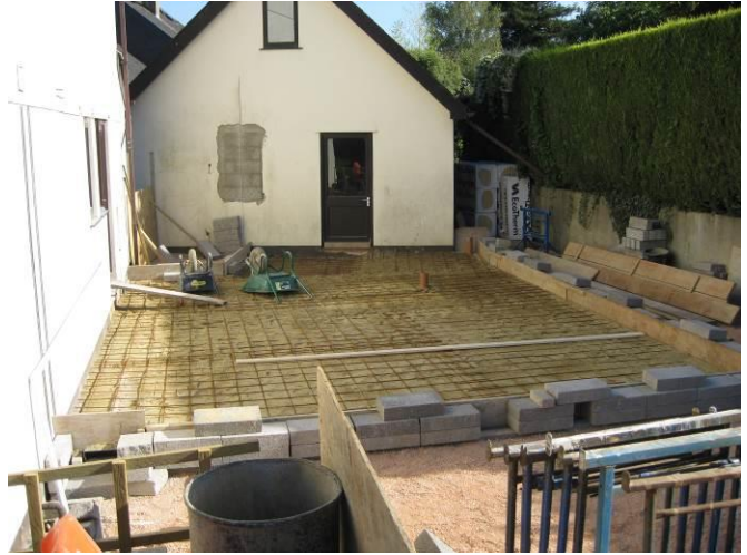
Reinforced Concrete Slab
