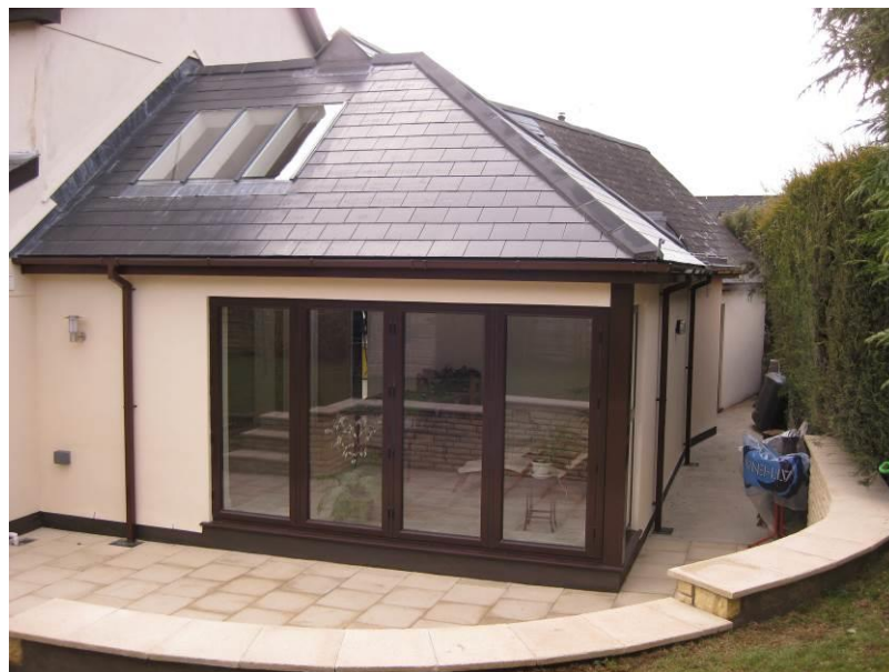
Rear elevation of extension
