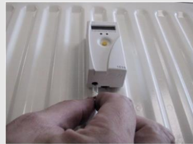
7-135 INSERTING THE SEAL
