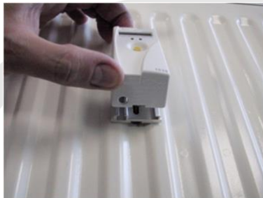
7-12 MOUNTING EHCA ON HEAT CONDUCTOR
