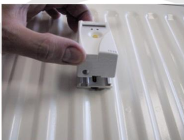
8-14 MOUNTING EHCA ON HEAT CONDUCTOR
