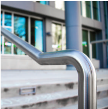
Single Line Handrail at Kansas State University
