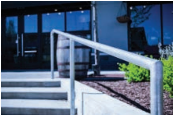
CARBON STEEL SINGLE LINE HANDRAIL
