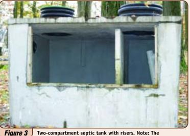
Two-compartment septic tank with risers. Note: The hole is for viewing purposes.
