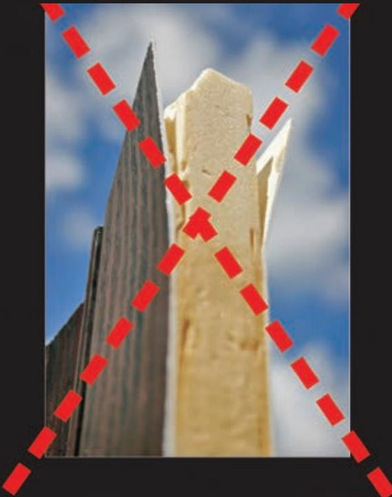
The picture above shows conventional composite doors, comprised of two 2mm skins bonded to a foam core.
