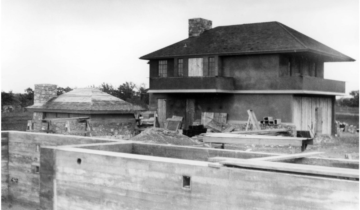
Graycliff under construction – July 5, 1927.
