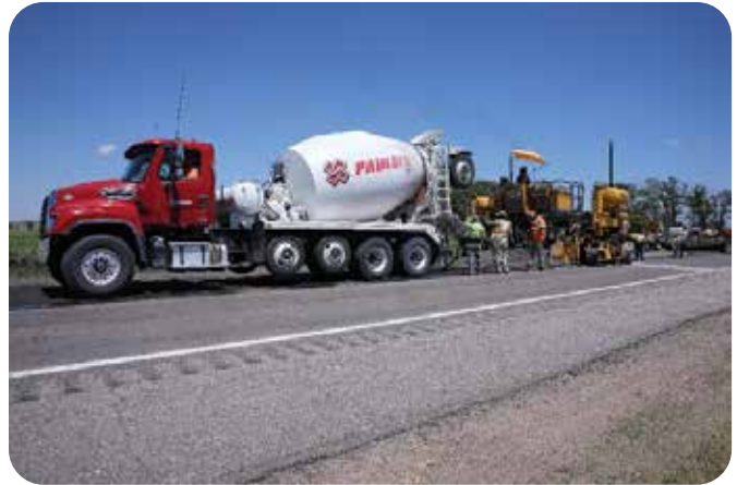
Paving and Redi-Mix paving between Brady and Maxwell.
