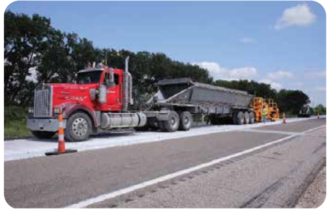
Asphalt paving the shoulders between Brady and Maxwell.
