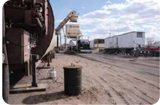
Asphalt Plant at Mills Loadout Area
