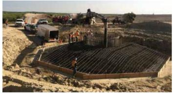
This is one of 43 bases we are pouring at the Broken Bow wind farm. Each base pour takes 324 cyds of concrete or 32 truckloads!
