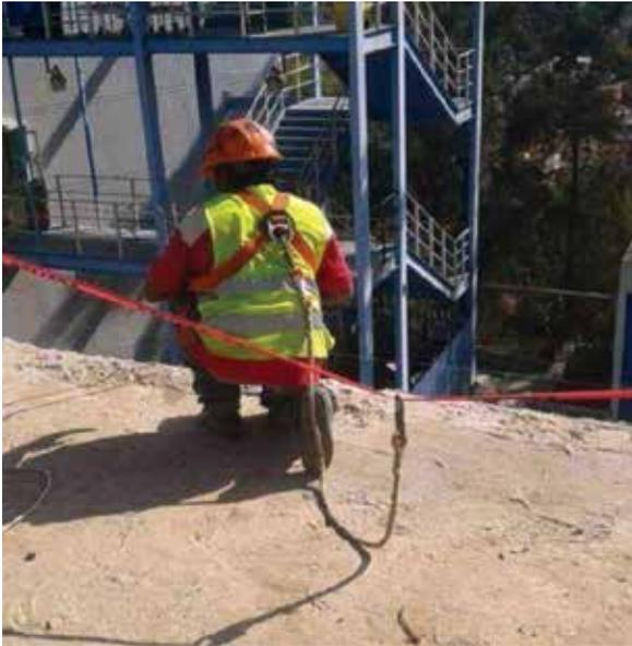
The harness might be OK, the lanyard looks OK but the anchorage point is barricade tape and I don't think it will support a pick-up truck!!!
