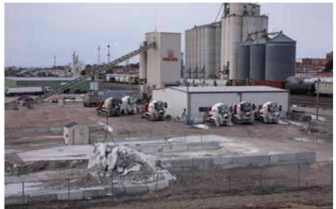
The McCook Plant
