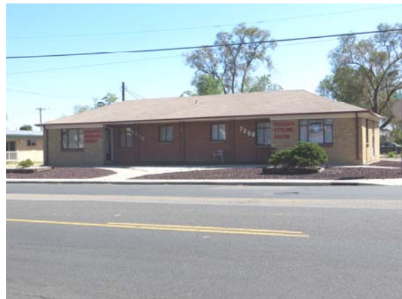
Figure IV-17. This duplex, accommodating a professional office and a beauty salon, is located at 7250-7260 Magnolia Street (5AM3169) and was built in 1951.
