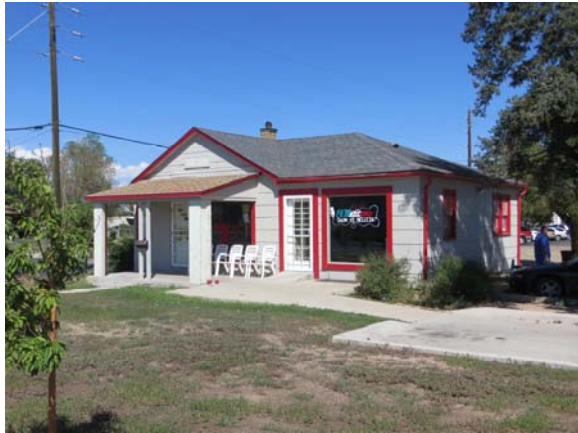
Figure V-6. Although altered for commercial purposes, this house at 6601 E. 72 nd Avenue (5AM3136) still retains its wood double-hung windows with upper sash containing divided lites.
