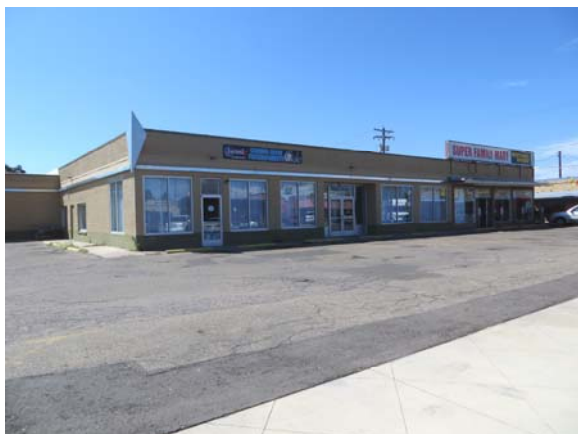
Figure IV-16. The Hi-Lo Market and Shopping Center Pharmacy earlier conducted business from 6470-6490 E. 72 nd Place (5AM3143), constructed in 1951.
