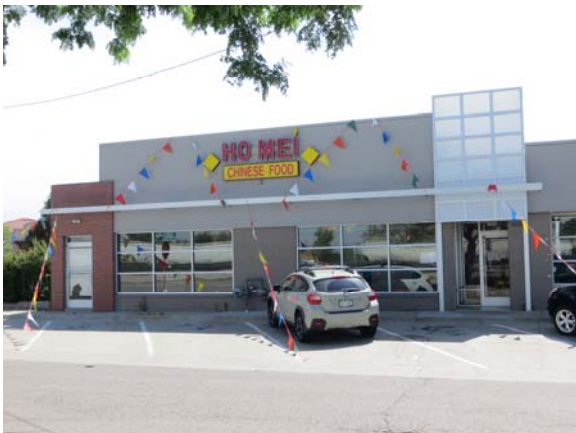
Figure V-11. 7270-7272 Locust Street was recently remodeled for a restaurant. Unfortunately, this resource and 7260 Locust Street have lost their Post-WW II features.
