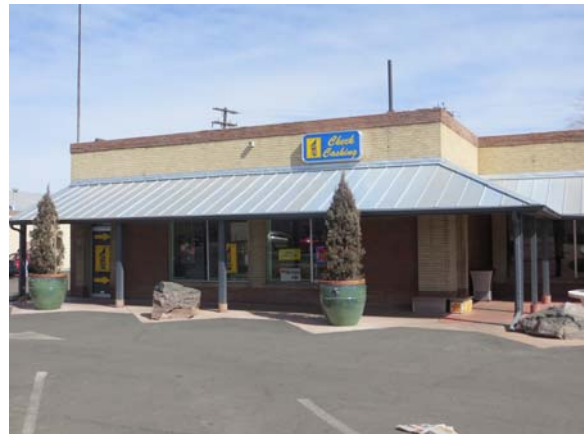
Figure IV-18. Adams County Assessor's records indicate that the north half of this strip shopping center, 7270-7280 Monaco Street (5AM3186 & 5AM3187), was constructed in 1952.
