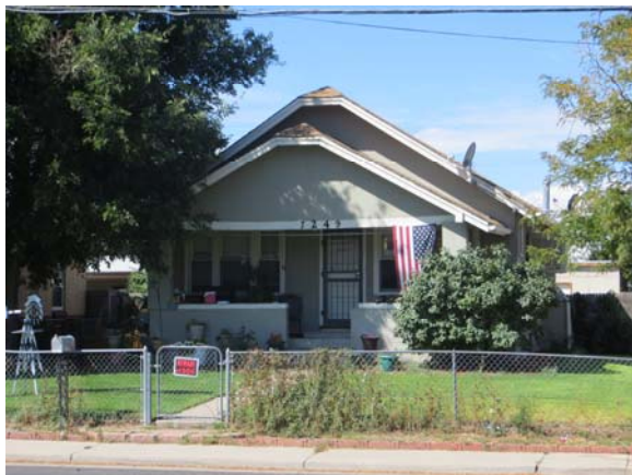
Figure V-7. The house at 7249 Magnolia (5AM3168) serves as a good example of the Craftsman Style with its low-pitched hip-on-gable roof, exposed rafter tails, decorative beams under the porch gable, and partial-width front porch.
