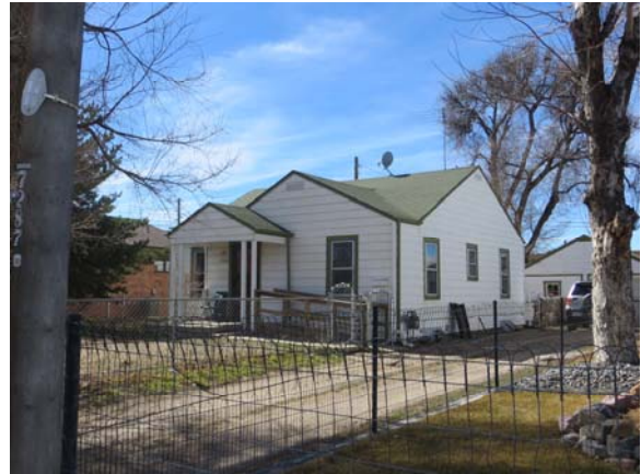
Figure V-8. This Minimal Traditional type house at 7261 Magnolia Street (5AM3172), constructed in 1945, incorporates a low-pitched front facing gable with close eaves and rakes.
