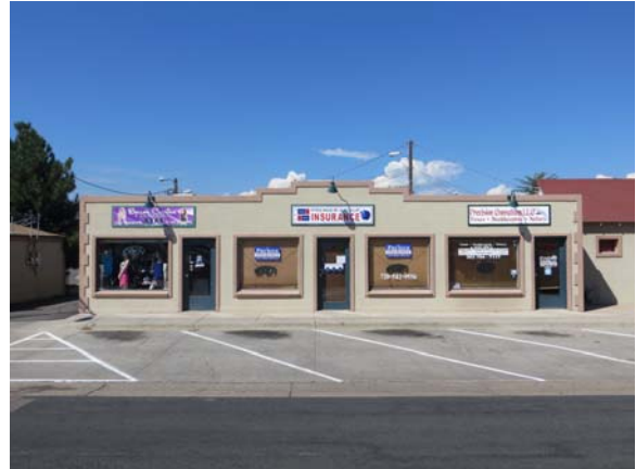
Figure V-4. This multi-tenant building at 7291-7295 Monaco Street (5AM3191) was built in 1957. The storefront windows and entry doors appear to be original historic building fabric but stucco was applied to the walls and former brick rowlock sills in 1988.
