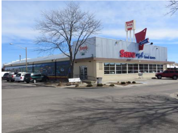
Figure V-2. The original windows at the Save a Lot Food Store at 7290 Monaco Street (5AM3190), constructed in 1953, were replaced. The new windows have wider frames to hold insulated glass and are oriented horizontally instead of vertically like the original units.
