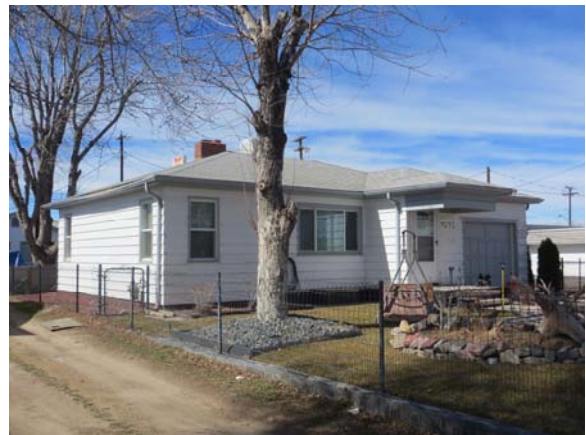
Figure V-9. The lack of decorative detailing and low slope roof at 7271 Magnolia Street (5AM3172), built circa 1953, are characteristics of the Minimal Traditional type house.
