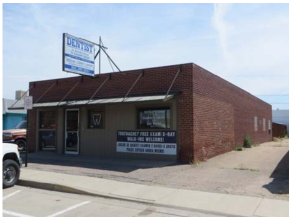
Figure IV-24. The Econo-O-Wash Laundry served Derby from this location at 7230 Locust Street (5AM3162) beginning in 1962. A portion of the original storefront was replaced with wood siding to accommodate a dentist's office.
