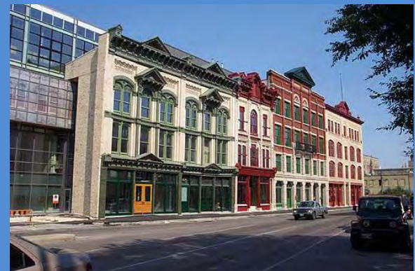
Red River College led an exciting new program downtown that restored 6 heritage façades in downtown Winnipeg.
