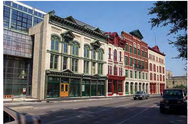
Red River College, was an exciting new program downtown that led to the restoration of 6 heritage facades
