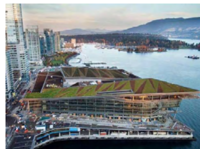
Vancouver Convention Centre is home to a 6 acre living roof containing 400,000 individual indigenous plants
