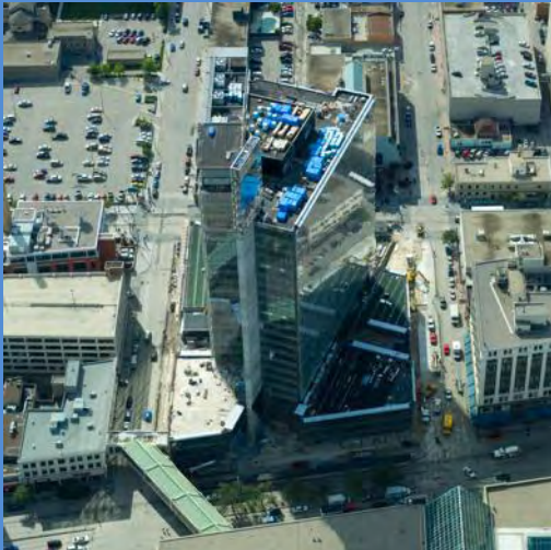
More than three-quarters of Winnipeg's office space is located downtown, among the highest proportions in Canadian downtowns. The new Manitoba Hydro Place is a prestigious addition to the downtown skyline.
