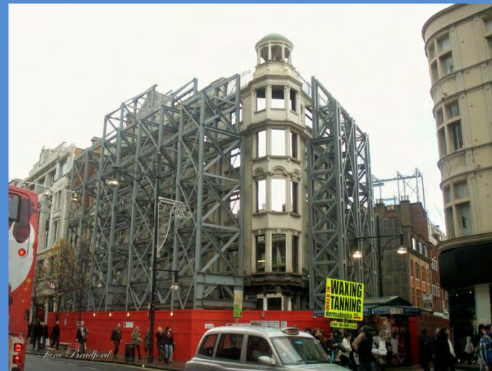
Example of building redevelopment, while preserving structural heritage. Oxford St, London, UK
