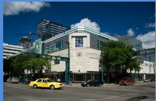
The University of Alberta's downtown campus in Edmonton occupies the renovated Hudson's Bay building, constructed in 1894.
