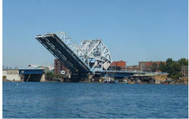
Johnson Street Bridge, 2010
