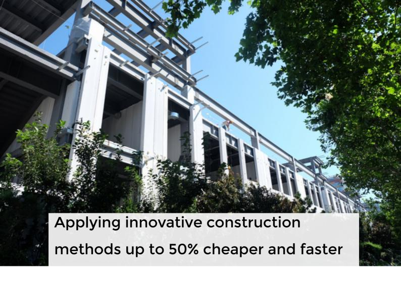
Construction methods: steel structure with prefabricated panels
