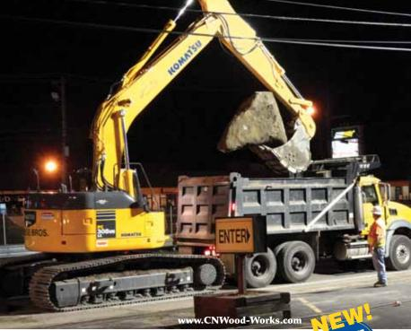
This Albanese operator uses the company's new Komatsu PC308 excavator on a sewer and water-line job in Saugus, Mass. "I love the tight-tail-swing PC308," said VP Oto Albanese. "It's great on road jobs because it's got good size but can swing safely with traffic in the next lane."
