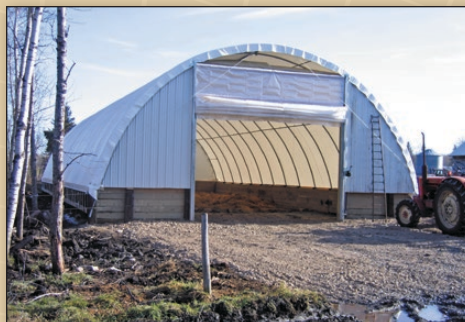
Our own polyethylene covered end wall provides a strong and attractive finish to your Diamond Shelter . End walls can also be wood or metal clad.
