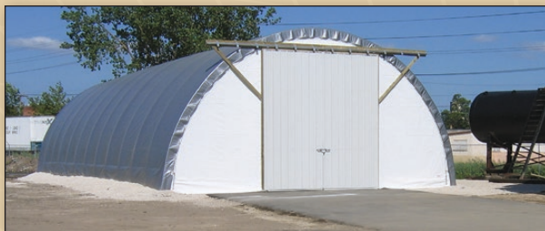
A beautifully finished 32' x 60' Freestanding Diamond Shelter used for storage.
