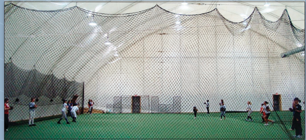
120' x 132' Freestanding Baseball Practice Facility
