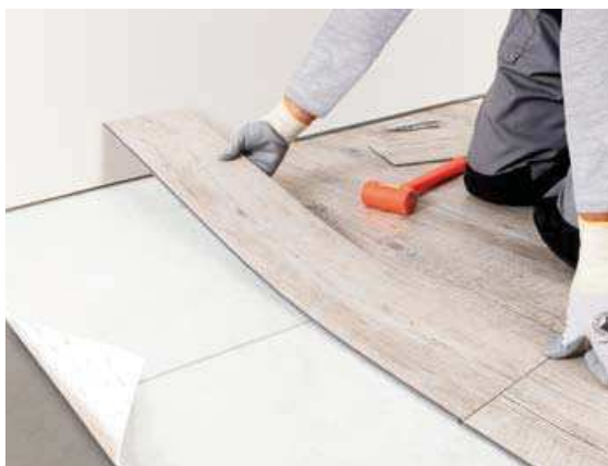
Possible installation on Gerflor underlayer for better sound insulation.
