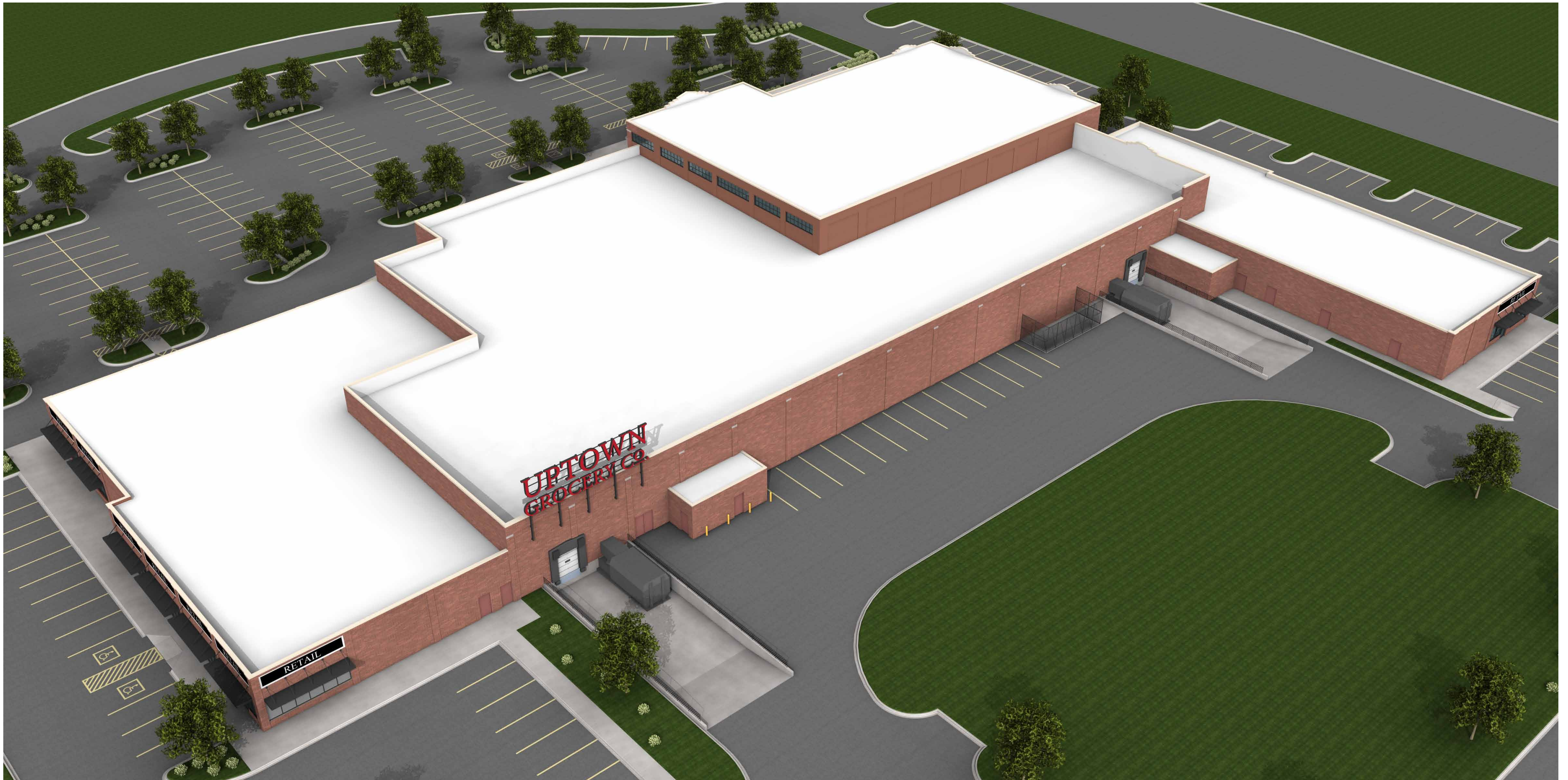
Aerial view from south-east
