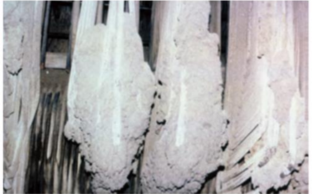
Slag on superheaters tubes ( www.boilers.guide )
