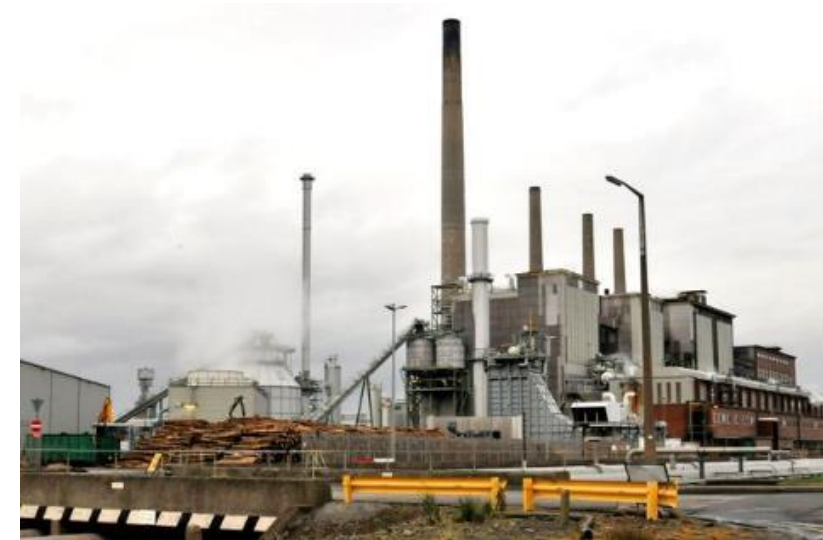
“Wilton 10” 35MW e Combined Heat & Power Station Bubbling fluidized bed Virgin wood + demolition wood blend
