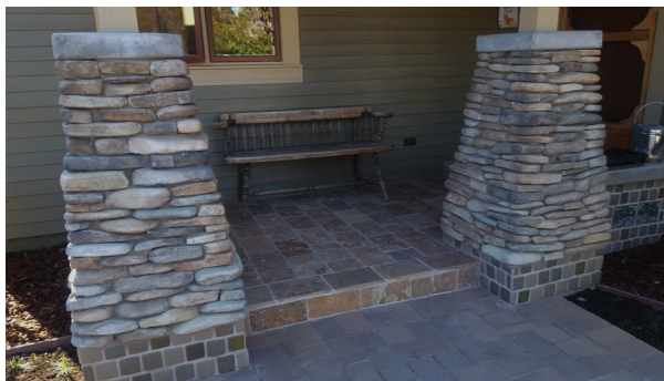
Figure 8. These column bases were crafted from local stones. Using local materials evokes our connection to nature. Private garden, Oceanside, California.
