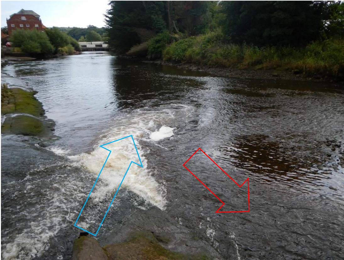
Figure 6. Looking d/s at the discharge from the baulk pass (blue arrow), creating a major attraction towards the baulk and, when the baulk is not passable, to the LB channel (red arrow). Note the wider, shallower, less attractive approach to the RB channel (far right of shot).
