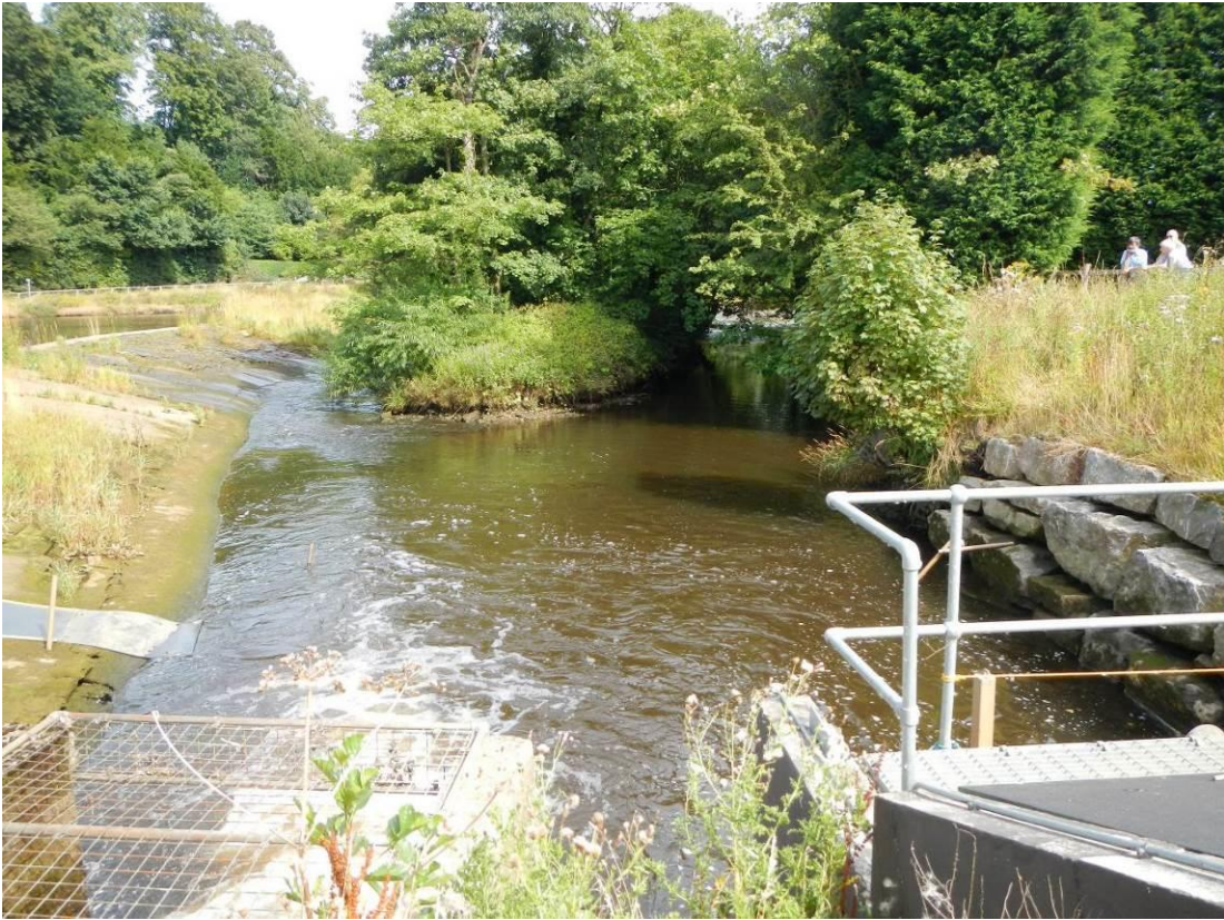
Figure 2. Larinier pass (foreground left) discharging flow that is then split down either side of the island (centre background). The hydropower installation (right of shot) was not in operation (or discharging) at the low flows observed. The proposed dredging would lower the RB channel (right of shot) and send a greater portion of flows down that channel.
