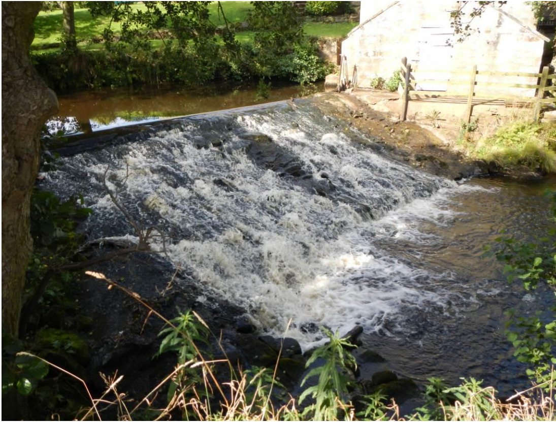
Figure 11. The height and steep c.100% slope makes Danby Weir a major barrier to fish passage severely inhibiting utilisation of spawning and juvenile habitat in the upper river.
