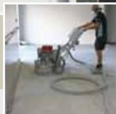
Preparing new floor for a meat processing plant and coating with SV100
