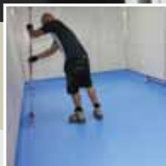
Preparing new floor for a meat processing plant and coating with SV100
