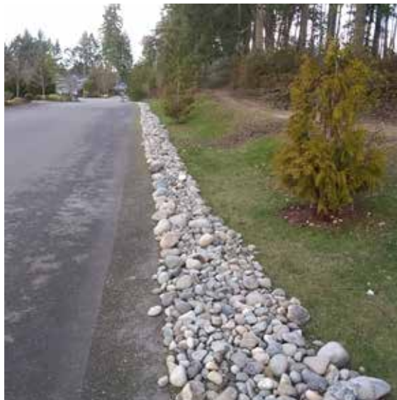
3. Whispering Pines Dr. had the hiking trail graded, boulders were added, and river rock was placed along the street edge to aid in drainage and slope control.
