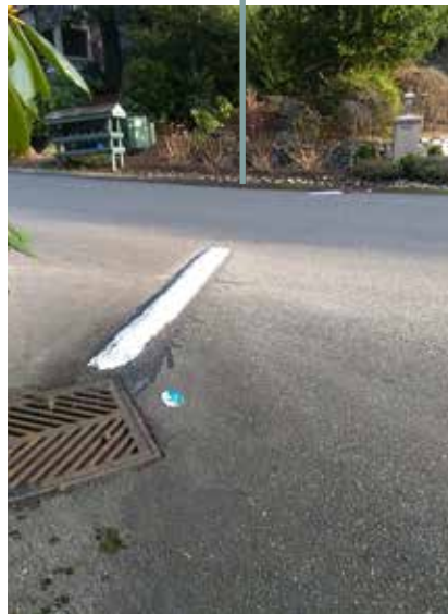
4. Along specific streets, drain bumps were installed and painted in order to be more visible for walkers, especially in dark conditions.
