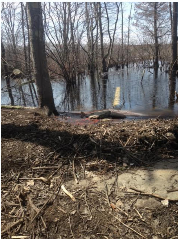
Pond leveler installed April 2017. Prior to the pipe and cage system installation, the dry land was all under water.
