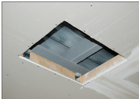
1. Wood frame installation
