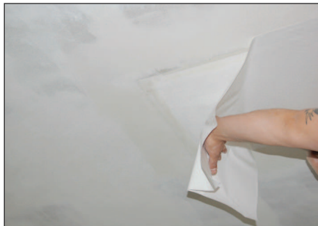
4. Application of the protective papersheet
