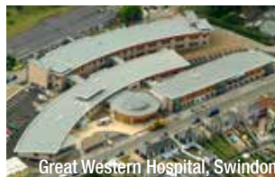
Great Western Hospital, Swindon
