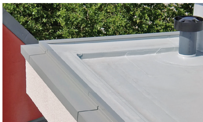
Installation over External Thermal Insulation Composite Systems (ETICS)
