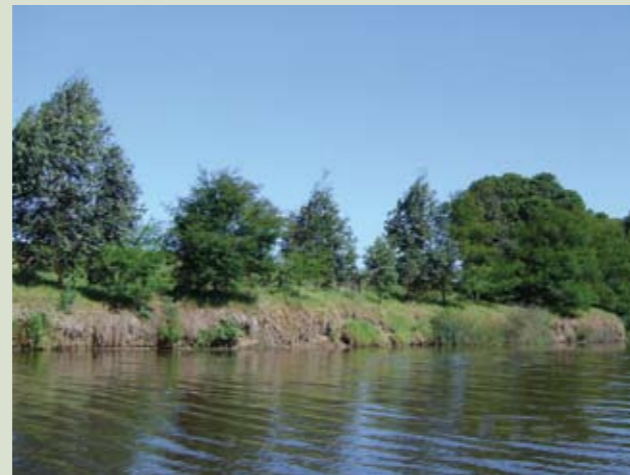
The same area in December 2004. The bank is severely undercut and has slumped. Revegetation began in spring 2001 and continues.
