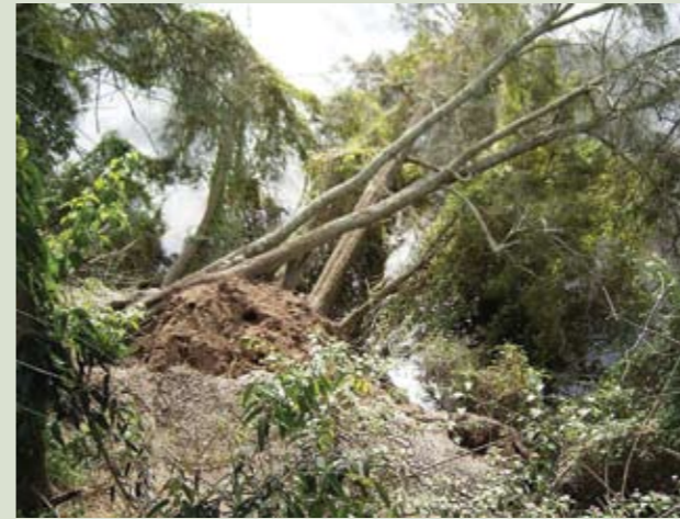
Severe erosion on the riverbank. This occurred on a straight section of riverbank after a river 'fresh' in June 2004. Riverbank restoration was integral to our whole farm plan.
