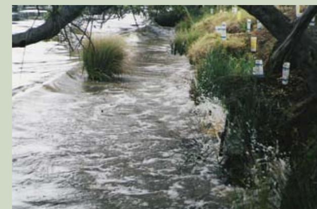
The destructive force of boat wash makes our efforts to plant protective vegetation difficult.
