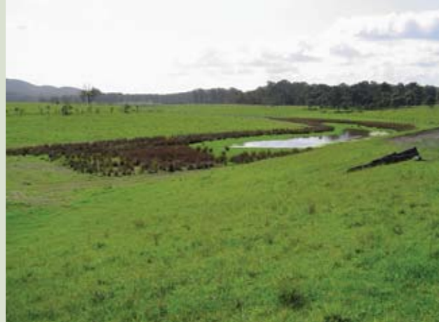
A lagoon wetland connects to the river via a drainage channel and floodgate. The wetland and channel has been fenced using two-strand electric wires and galvanized star pickets.
