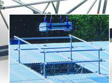
Supply of building materials from above: at any point on the roof cassettes can be removed for pinpointed material supply.
