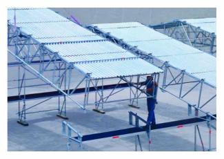
The girders are connected and stiffened on the ground, the roof cassettes placed on them, and the finished unit is lifted by crane onto the supporting scaffolding. Only every second roof bay is assembled as a complete truss. That saves on materials and assembly time.
