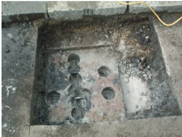
Cover meter survey & rebar exposures in trial pit to confirm outer corner bars on portal frame.
