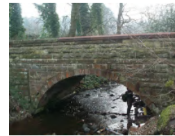
Masonry bridge investigation
