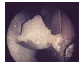
Bore scope inspection of wall ties.
