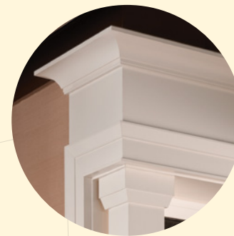
The architrave is always deeper than the corresponding Scene casing, ensuring a proper reveal at the joint.
