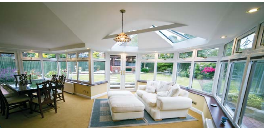
LivinROOF replacement project
