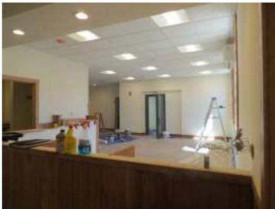
Interior under Construction
