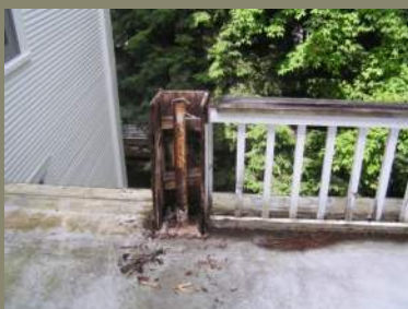
Existing Railing Conditions
