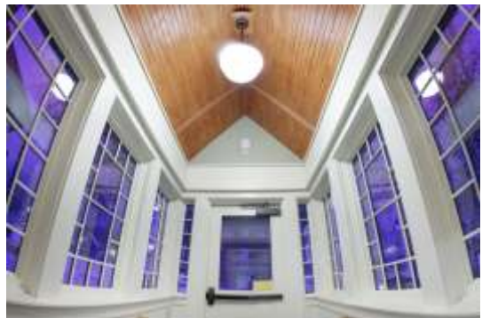
New Side Entry to Offices
