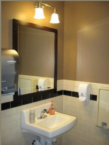
Interior Bath Renovation
