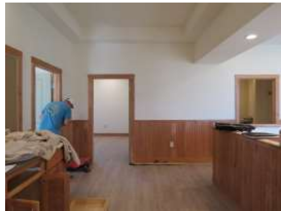
Interior under Construction
