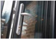
Please note the lever handle option is not an anodised product and will not be suitable for coastal applications
