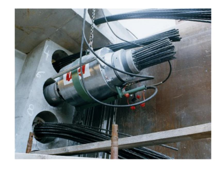
The hydraulic jacks used to tension the post-tensioning tendons range from compact 60 lb jacks used to stress monostrand tendons and small bar tendons, to very large jacks requiring special hoisting equipment, used to simultaneously tension all of the strands in large multistrand tendons.
