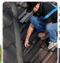
1. Cut along the ridge of the tile. The mesh will sit on the top of the tile against the ridge of the tile.
