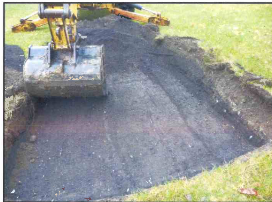
Image 86: Surface of Cinder Layer Exposed in Grid 5 Western Anomaly Investigation Area (looking east)
