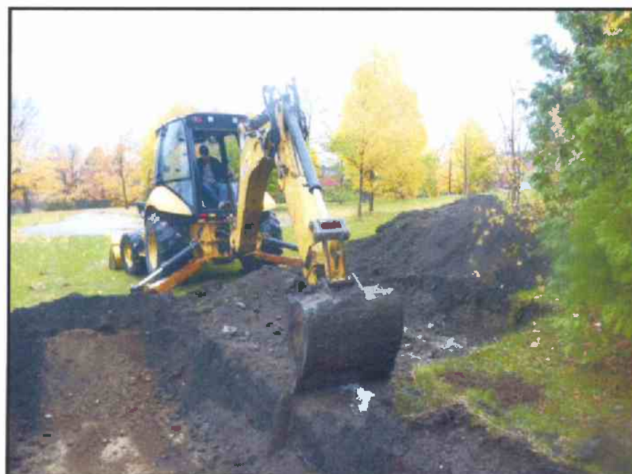
Image 89: Exposing Asphalt Walkway in Grid 5 Western Anomaly Investigation Area (looking east)
