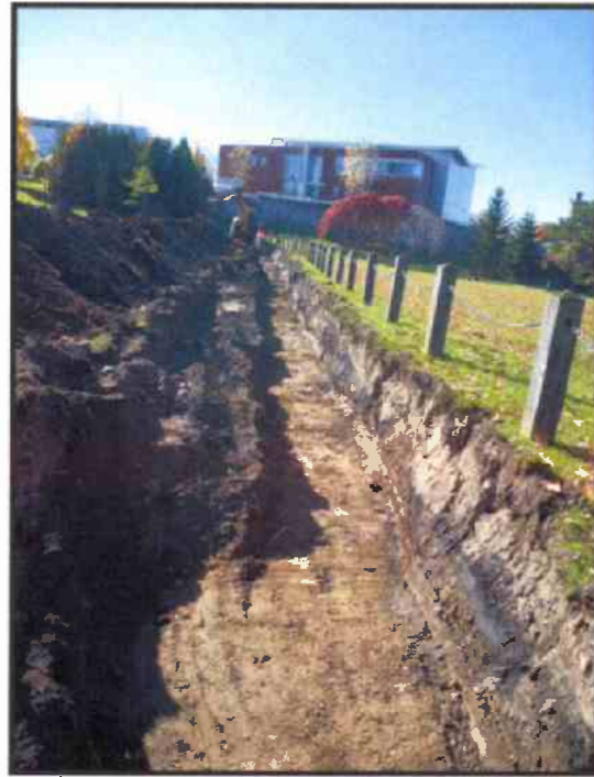
Image 67: South Trench Excavation (looking west)
