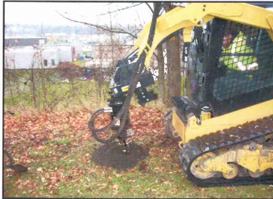
Image 97: Post Hole Augering for New Fence (looking north)
