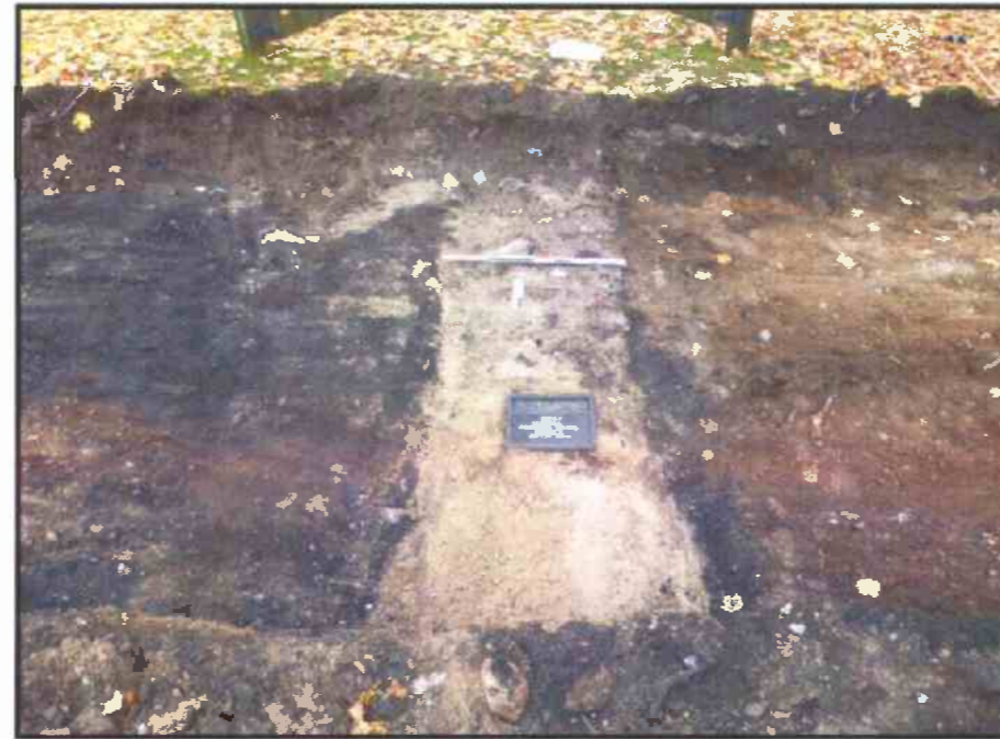
Image 68: Buried Culvert Beneath Existing Entrance Near Gate Along South Boundary (looking north)
