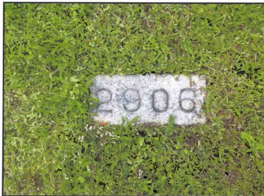
Image 16: Example of a Flat Marker with Stamped Registration Number (looking down and to the west)
