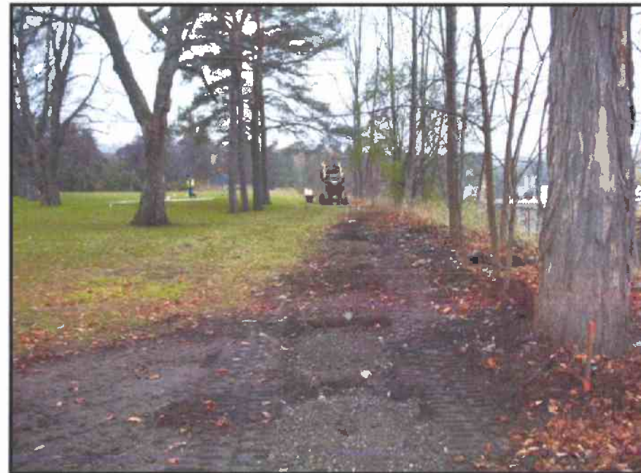
Image 98: New Post Holes on North End of Cemetery (looking west)
