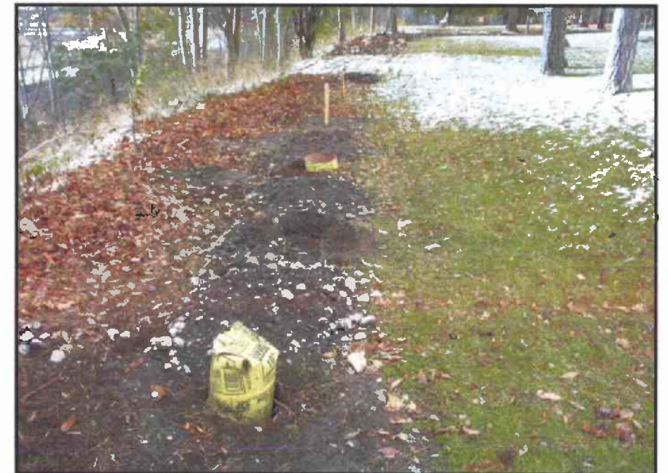
Image 99: Geotube Installation for Post Foundations - North Boundary (looking east)
