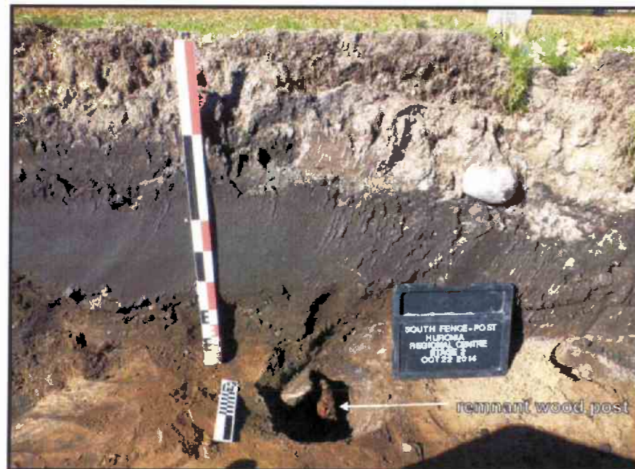
Image 70: Remnant Wood Post Identified in South Boundary Trench (looking north)
