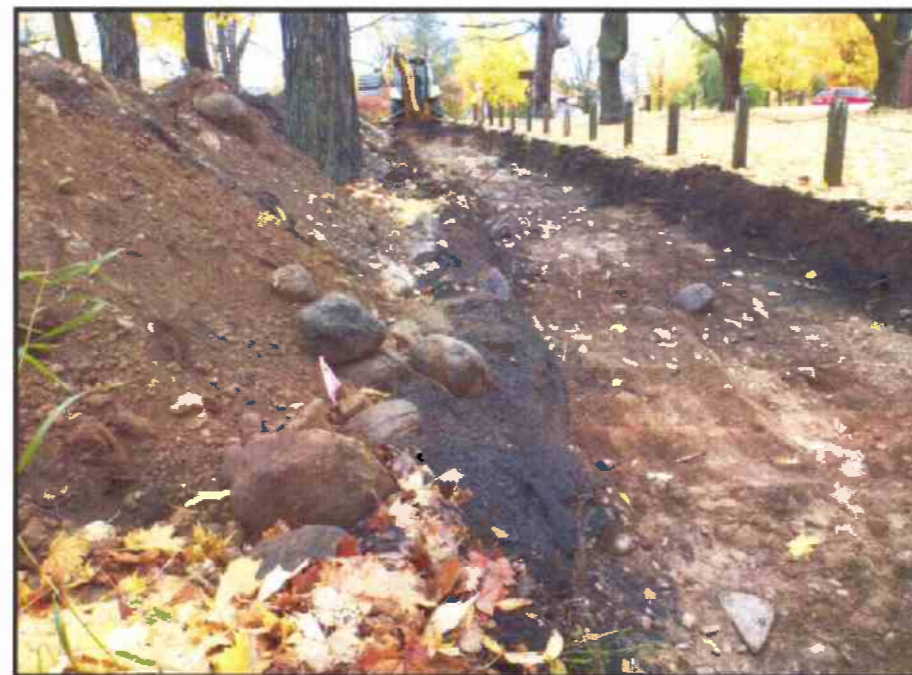
Image 62: Topsoil Stripping Along East Boundary in Progress (looking south)
