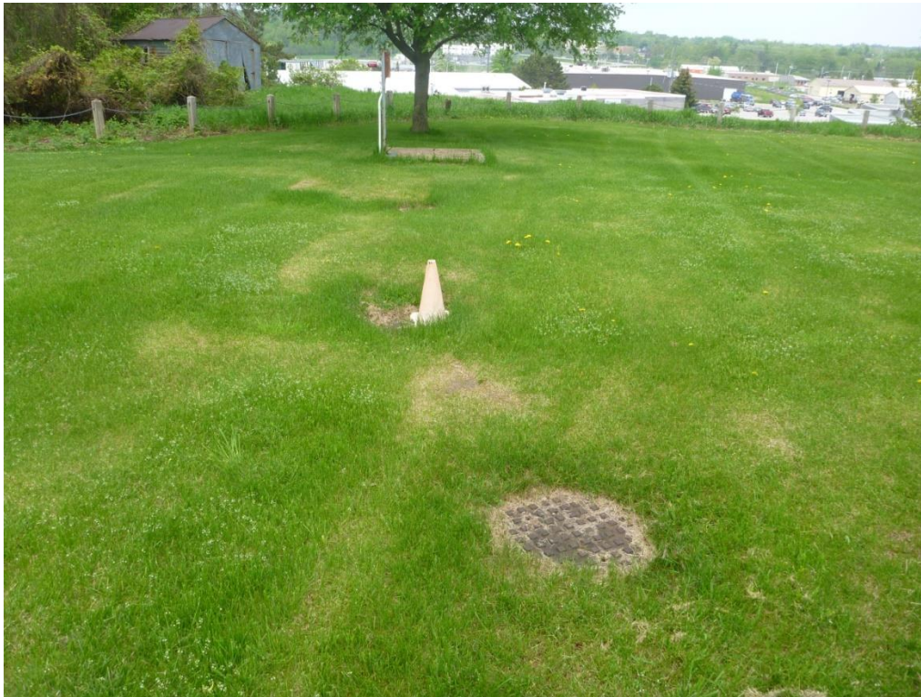
Photograph 1: Overview of Utilities Within the Cemetery Fence (looking northwest)
