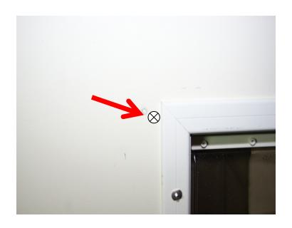
3) REMOVE THE DOOR AND DRILL THE CORRECT SIZE HOLE WHERE MARKED. THE SIZE OF THE HOLE WILL CHANGE BASED ON APPLICATION OF FASTENERS.
