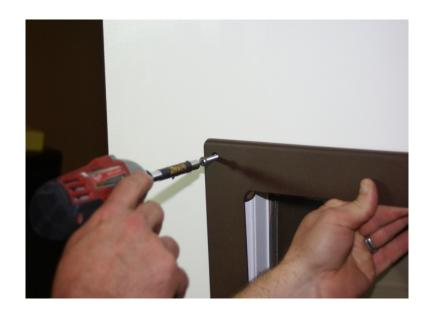
5) LEVEL THE DOOR AND REPEAT STEPS TO MARK, DRILL & TEMPORARILY INSTALL UPPER CORNERS WITH TAMPER RESISTANT SCREWS. NOW MARK BOTH BOTTOM HOLES, REMOVE DOOR, AND DRILL THE BOTTOM TWO HOLES. YOU ARE NOW READY TO INSTALL THE FRAME. FIRMLY TIGHTEN THE SCREW HARDWARE TO COMPLETE THE INSTALLATION.
