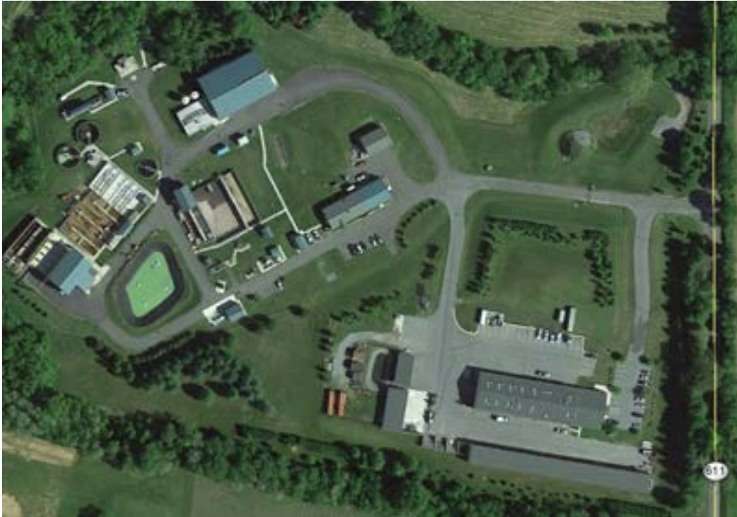
FIGURE 12: BASHAM SIMMS WASTEWATER FACILITY
