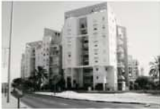
Fig. 8 Typical street front in the Israeli city
