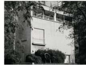
Fig. 9 Zacks Residence, Dov Karmi Architect, 13 Ben Gurion Bd., 1954
