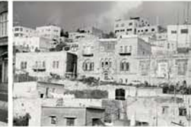
Fig. 6 Architecture without architects, Hebron
