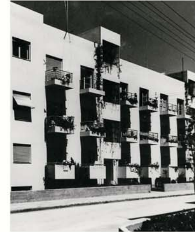
Fig. 12 Street front, workers' residences
