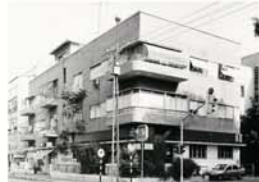
Fig. 7 Ripstein Residence, Sherkini St., 1934
