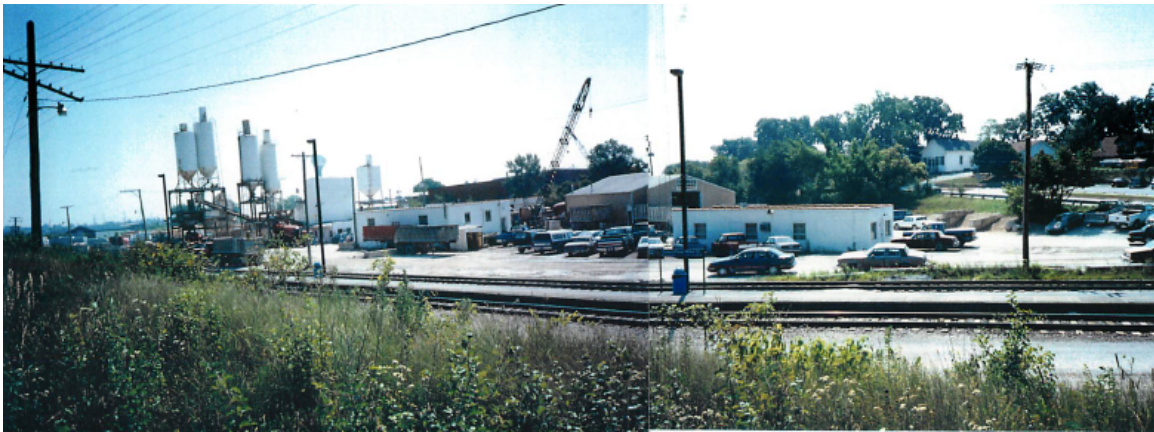
Davidson Concrete across the tracks from the train station.
